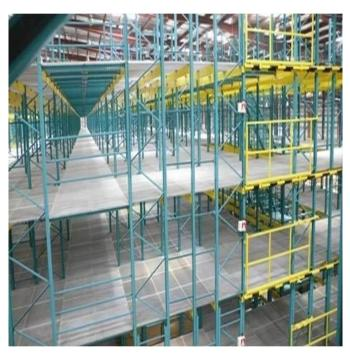
Frame based Mezzanine floors, also known as "rack supported mezzanines" are versatile systems which serve dual purpose of shelving space on ground and flooring space on top. Besides in a frame based mezzanine floor, you have the flexibility of defining your storage and aisle spaces.
